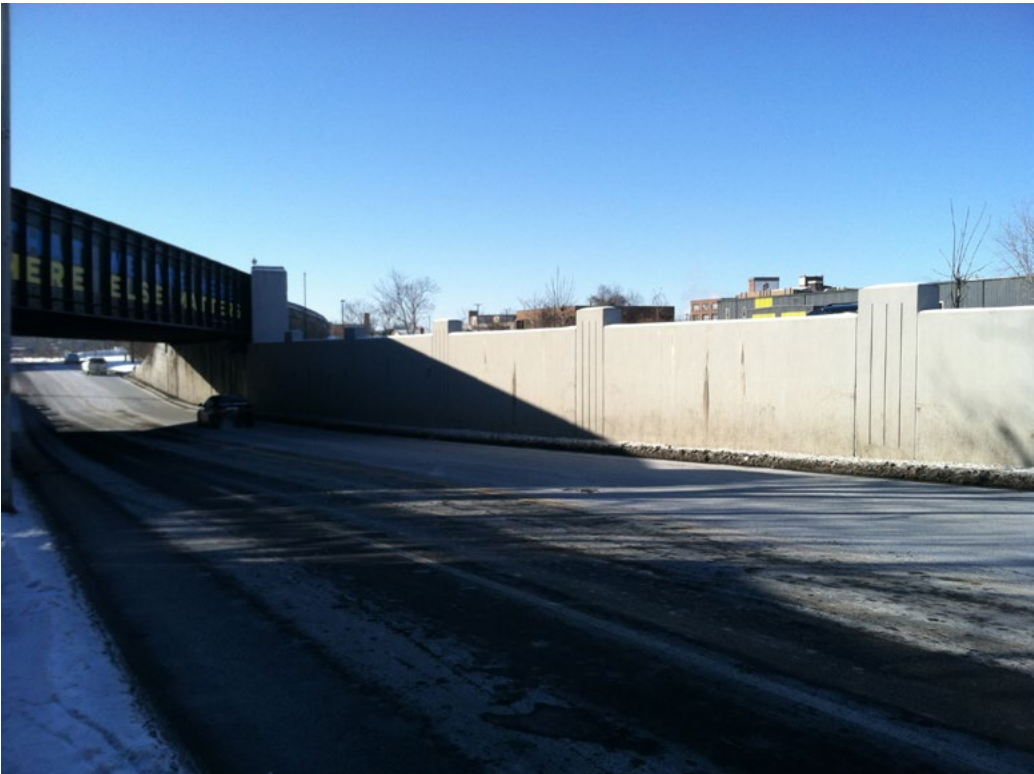
1b - Fayette Street Rail Bridge Underpass
