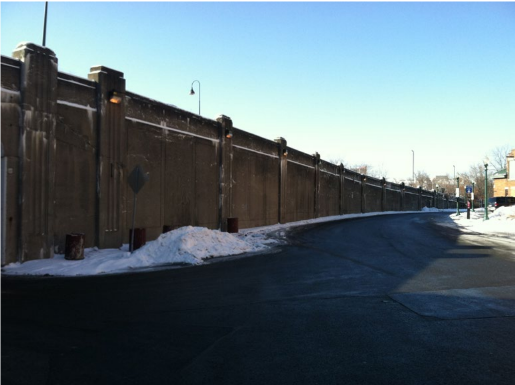
2 - Jefferson Street Wall
